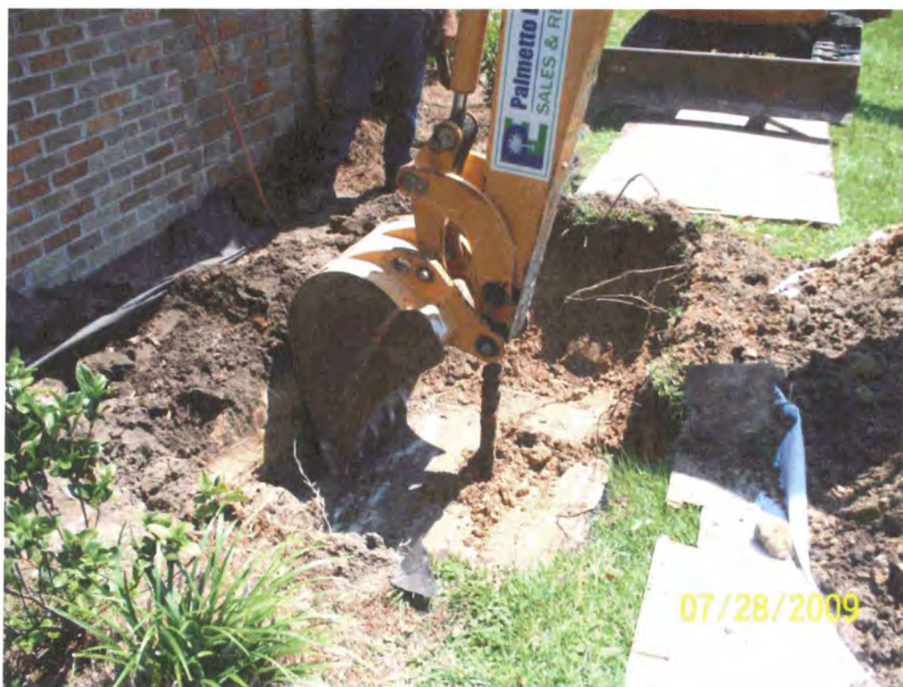
Picture 2: Removal of concrete lid over UST 1407Eagle-1
